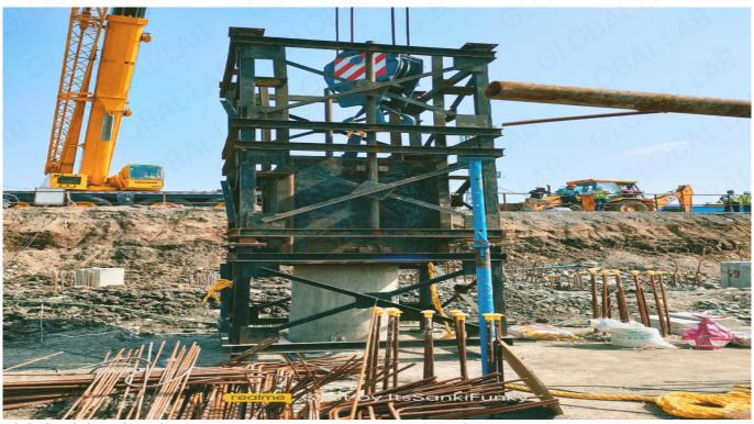
Global Lab has the Pile Dynamic Test as per ASTM D 4945 under scope of NABL.
